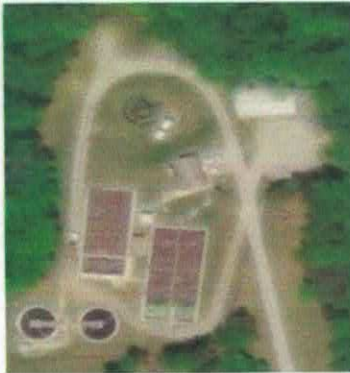
Town of Boiling Springs WWTP
